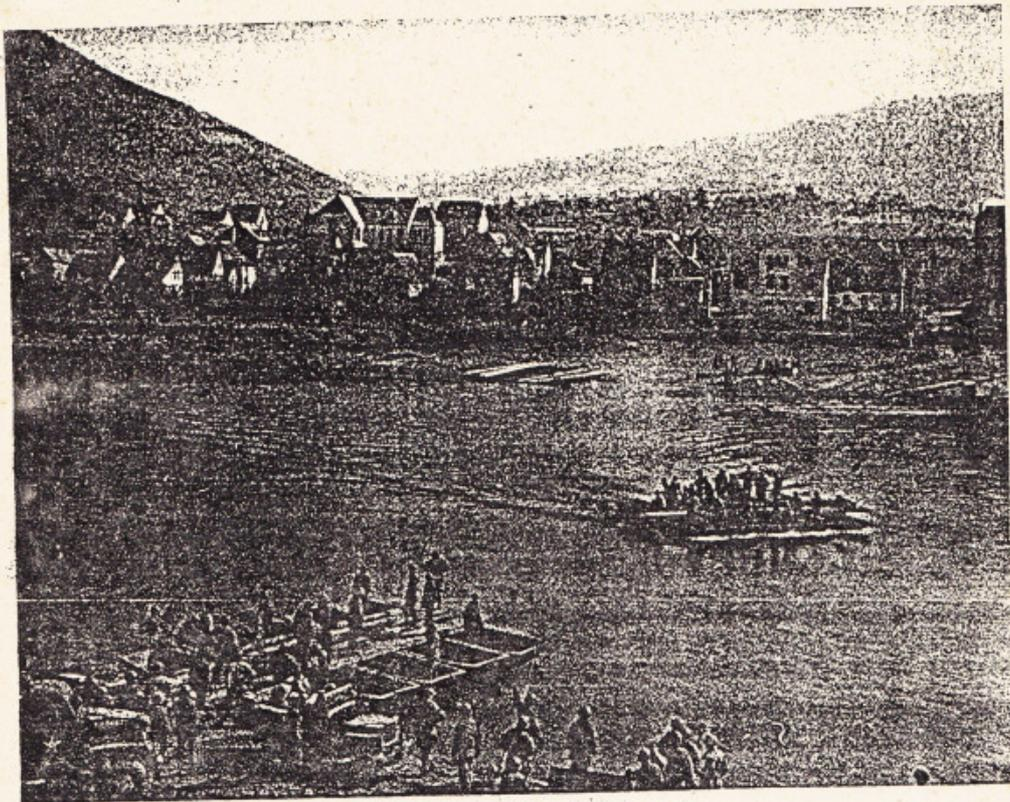
Engineers maneuver the second span of a treadway bridge on the Moselle between Alf and Bulloy.
